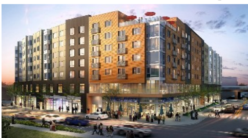
Centric apartments/retail building at the Little Italy-Mayfield Red Line rail station.
