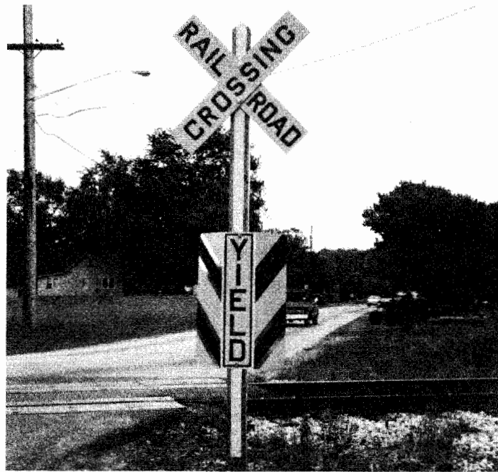
The new red and white reflective Buckeye Crossbuck , to be tested in Ohio, seen at the Fairchild Avenue crossing of the W&LE RR in Kent.
