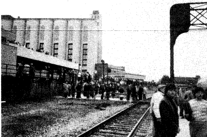
Former silos which have been converted into Akron's Hilton Hotel at Quaker Square, site of our March 23 meeting -- in the foreground the walkway leading to the Amtrak platform.
